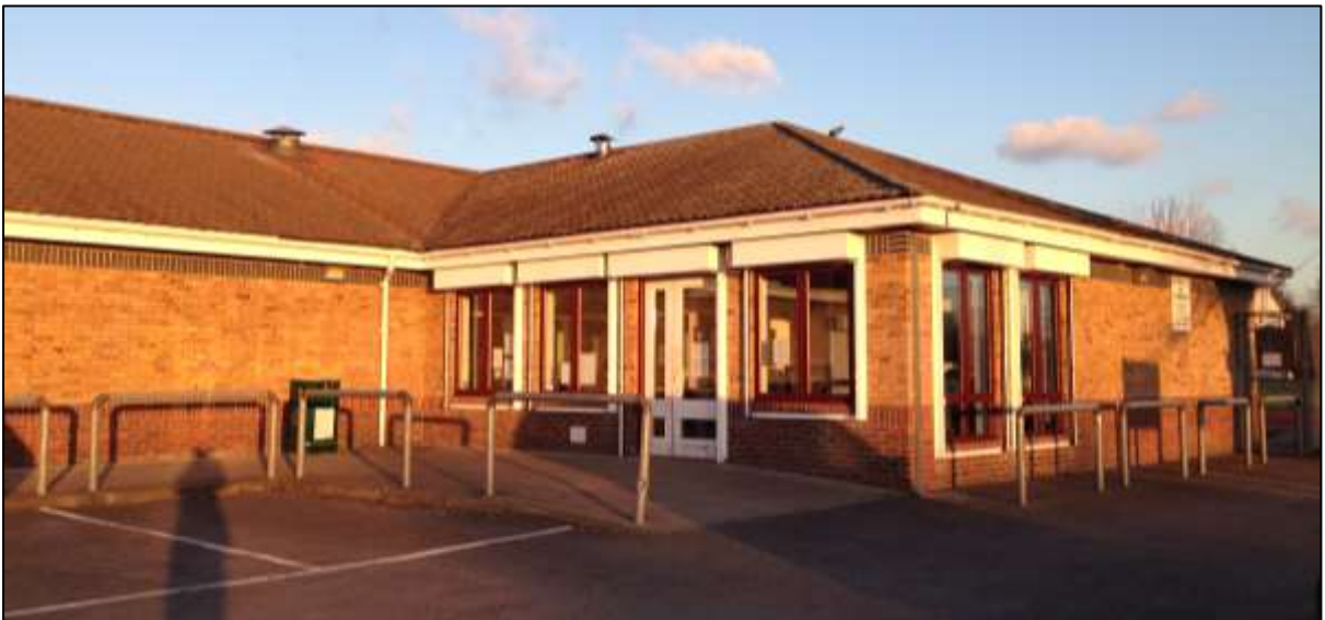
Figure 17 Pictures showing The Harrier Centre with access compliant with the disability discrimination act 1995
